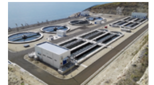
Sewage treatment plant
