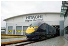
Ashford Train Maintenance Centre
