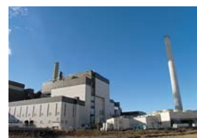
Walter Scott, Jr. Energy Center Unit 4
